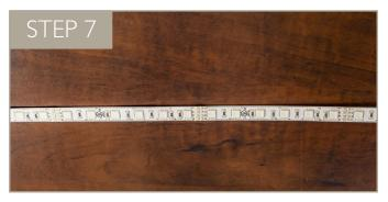
Carefully press the LED tape to the mounting surface. Secure lead wire from connector.
