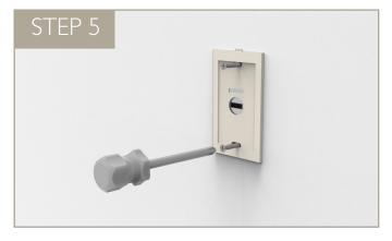
Secure wall mount controller base to wall box using screws provided.
